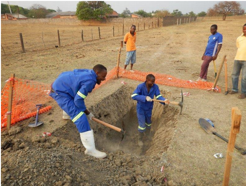
Excavation of pit for effluent (1)
