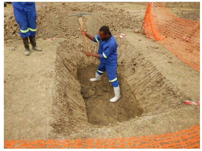
Excavation of pit for effluent (2)
