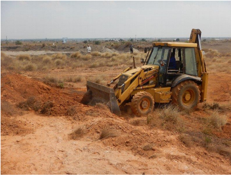
Excavation of Tailings from Kabwe
